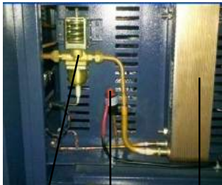
Water flow regulator Resetttable pressure switch Brazed Plate exchanger (water-cooled condenser)
